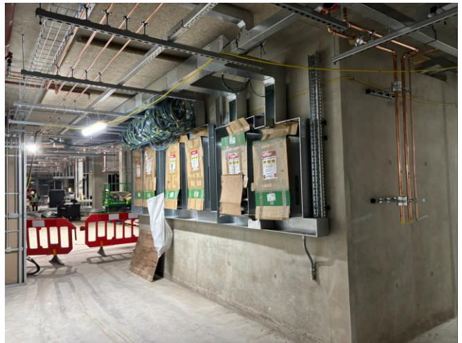
Electrical works in Zone 1, Level 1
