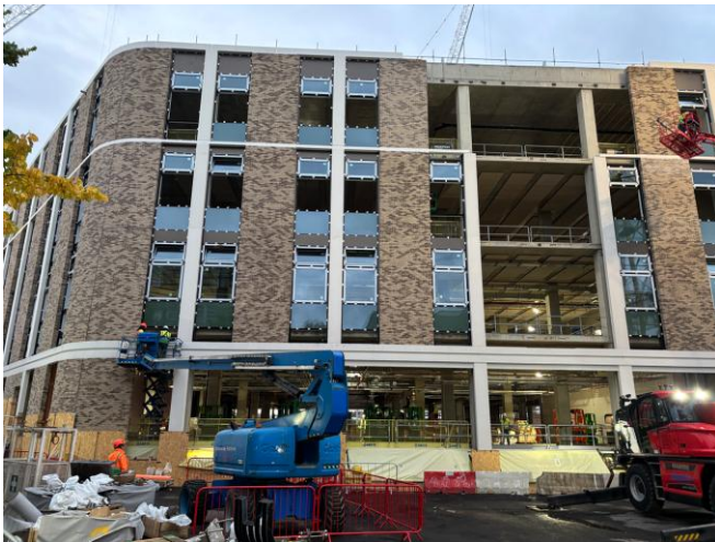
Glazing to North Elevation
