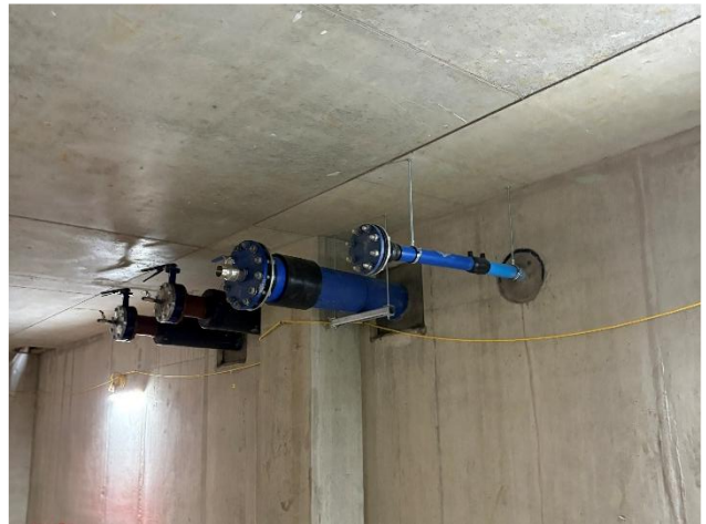
New building services entering the building
