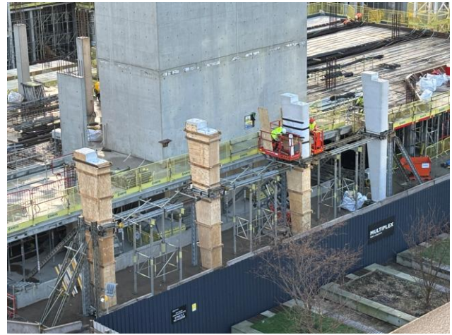
The next set of pre-cast columns are currently being installed
