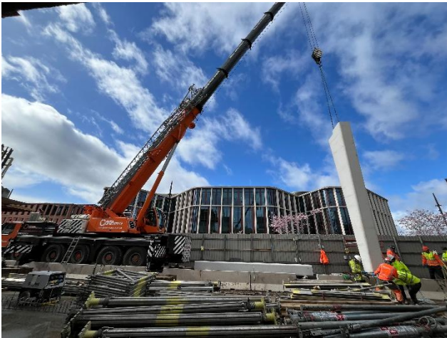
The next set of pre-cast columns are currently being installed
