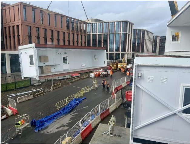
Additional cabins being installed
