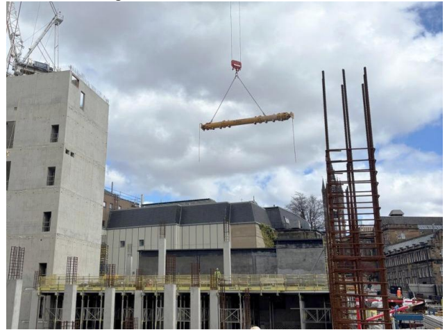
The final temporary prop being lifted out
