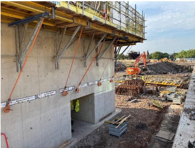
The first core walls have been cast
