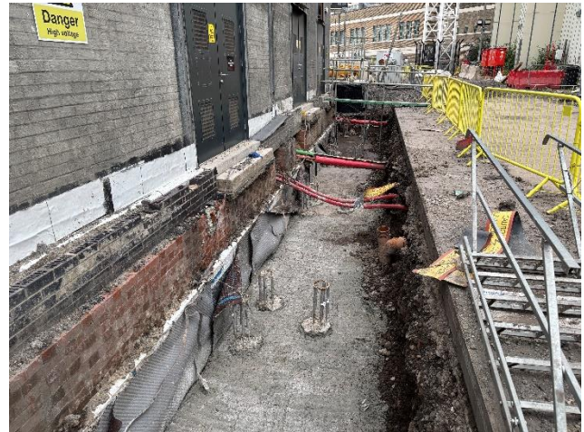
Excavation around the HV switchroom
