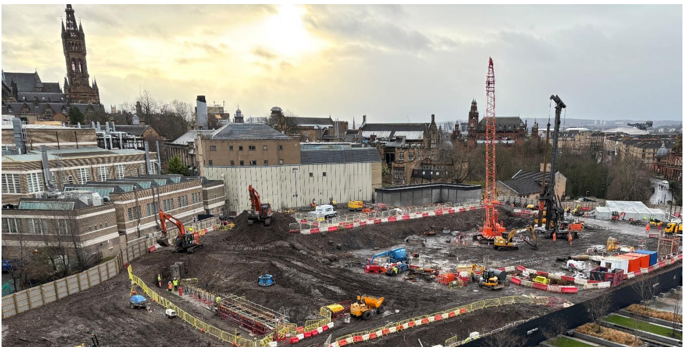
Aerial view of the site
