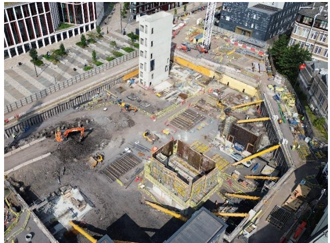
Extent of the basement from drone footage
