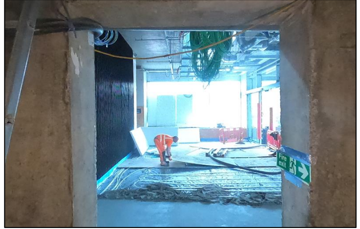
Weatherproofing complete and screed installation L1
