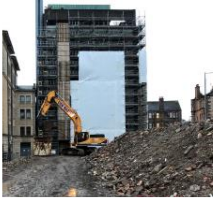
Pontecorvo Building wrapped ahead of demolition
